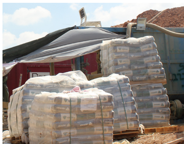
Bardala Bypass Pipeline construction site. Photo: Who Profits | 18.6.19
