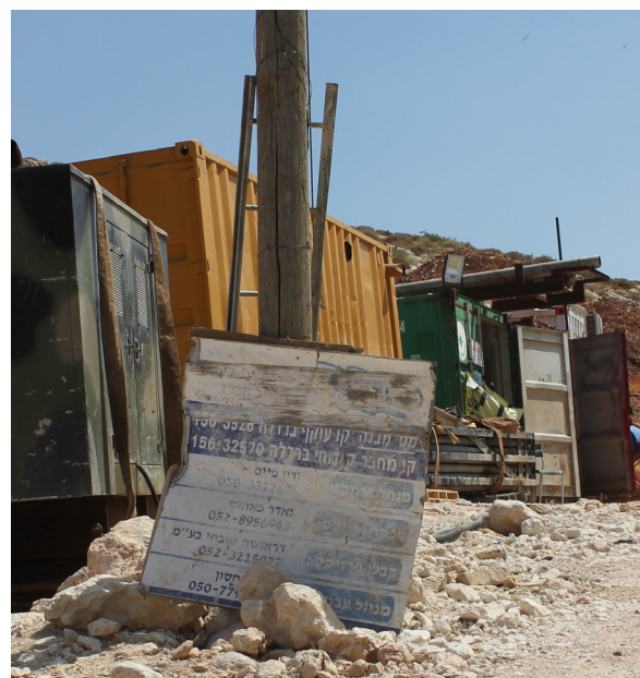
Bardala Bypass Pipeline construction site.
